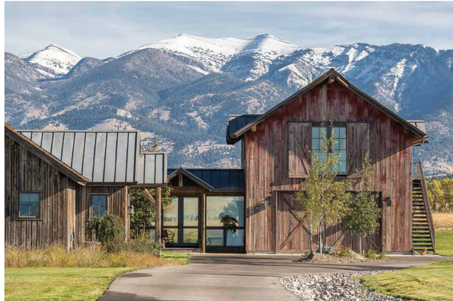
The red barn, crafted from reclaimed wood, references the architectural history of the valley and conceals an apartment and garage. The boards were strategically placed to look as if they had aged over the decades. The barn is connected to the home by a glass breezeway, referencing the transition from old to new.
